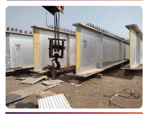
LC 112A: Railway Span Steel Girder Assembly work
