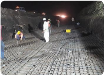
LC 115: Retaining wall raft reinforcement Route: Akola - Nanded Highway Section: Manmad - Mudkhed Location: Between Washim and Kekatumarg Stations
