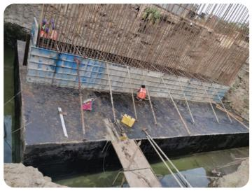
LC 122: First lift shuttering completed & first layer coal tar epoxy coating work
