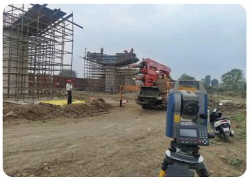
LC 290: Shuttering of Pier Cap Route: Road joining to Dahegaon village Section: Amla - Nagpur Location: Bharatwada and Kalmeshwar Stations
