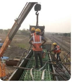
LC 136: Concreting for Pier cap Route: Amalner - Chopda Road Section: Udhana - Jalgaon Location: Between Amalner and Takarkhede Stations
