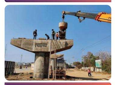
LC 144B: P13 Pedestal concreting work completed Route: Hingoli - Nanded Highway Section: Manmad - Mudkhed Location: Between Hingoli Deccan and Dhamani Stations
