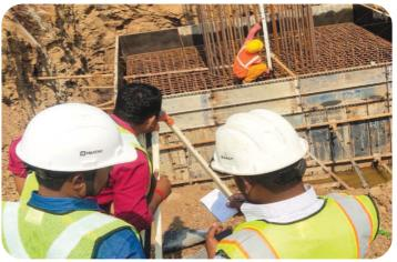
LC 20: Level Checking of Pier and Pier Cap
