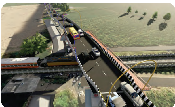
LC 119 Between Bhilwadi and Nandre station on Pune-Miraj Section of CR
