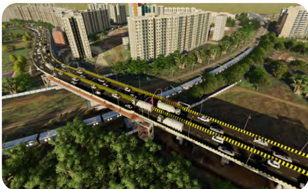
Titwala ROB (MMRDA) between Titwala and Khadavli stations on Kalyan-Igatpuri Section of CR
