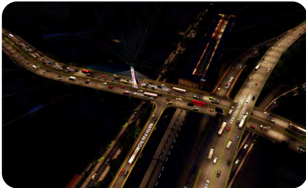
Night View of Cable Stayed Bridge at Byculla, Mumbai between Byculla & Sandhurst Road Railway Stations
